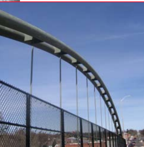
Ravenna, Neb., is home to the nation’s first post-tensioned, tied arch bridge, a UNL-patented design.
