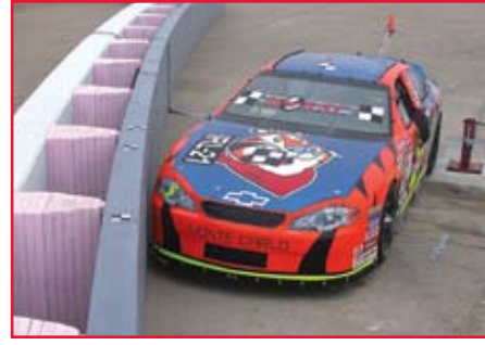
The UNL-developed Steel and Foam Energy Reduction (SAFER) Barrier protects NASCAR and Indy Racing League drivers.
